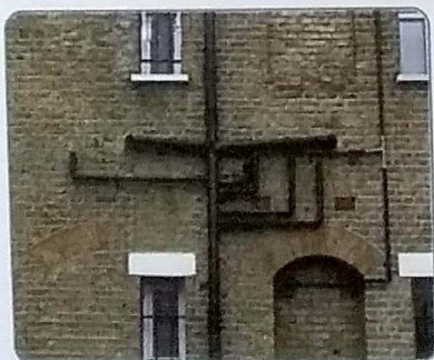
Proper drainage system
